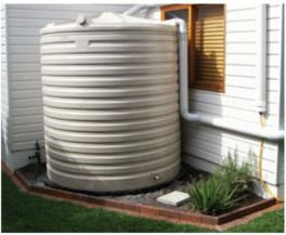
"Crusher dust" is available from nursery suppliers and is a mix of small crushed rock and fines. When compacted it binds together tightly creating a strong, stable surface for placing your tank. The crusher dust must be boxed in with some sort of retaining structure (e.g. retaining beams, bricks) to prevent it washing away over time.
